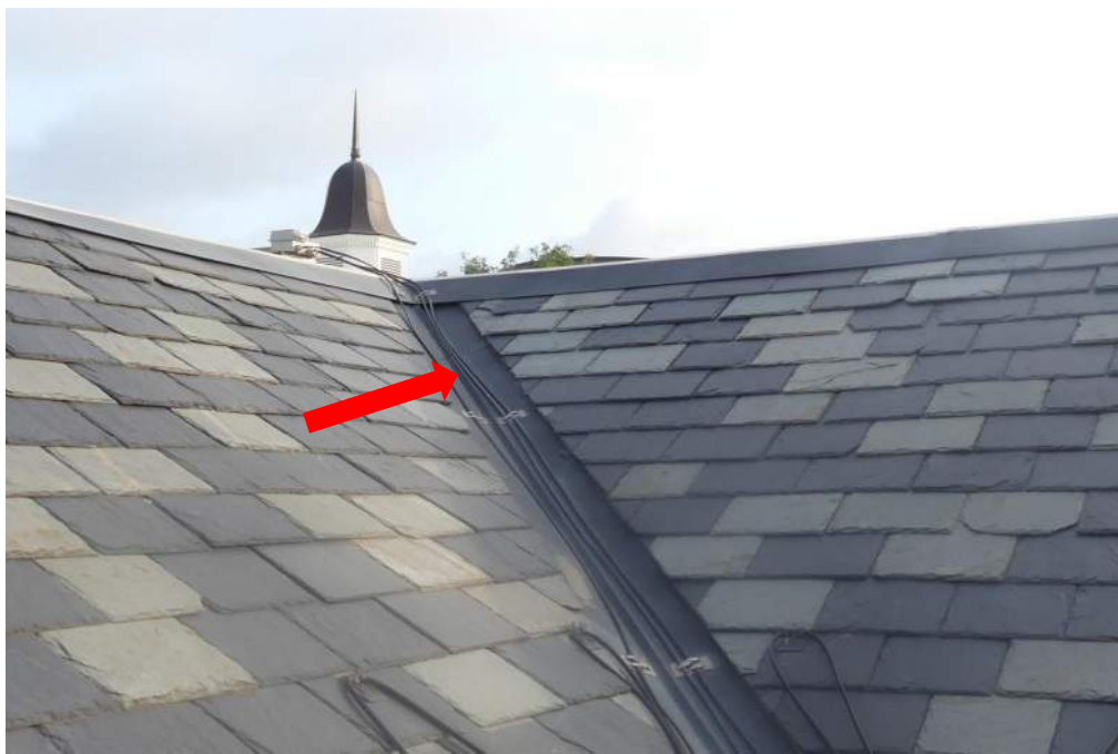
Photo 2 – The cables extended up the valleys located above the south entrance.
