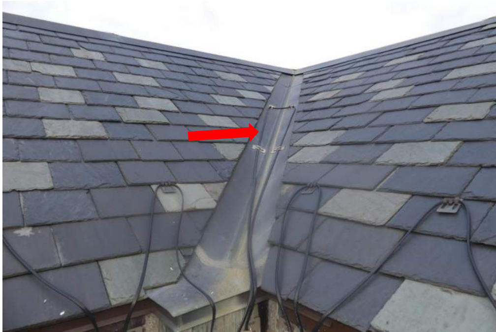
Photo 1 – The cables extended up the valleys located above the south entrance.
